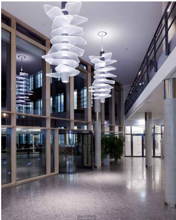
LED-Beleuchtung im Fraunhofer-Institut in Jena (Fraunhofer IOF).
